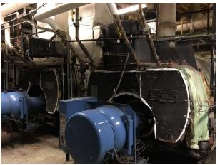
The Main Street campus is heated by two hot water boilers installed when the building was built in 1958. The boiler shells have had multiple crack repairs over the last few years.
