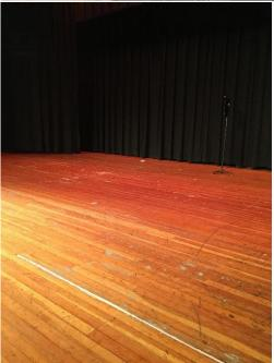
The current auditorium wood stage is too thin to refinish. The current cracks have been patched for several years in order to keep the surface safe. The current stage curtains will need to be removed in 2019 when the current fire retardant certificate expires. They are not able to be re-treated due to their poor condition.
